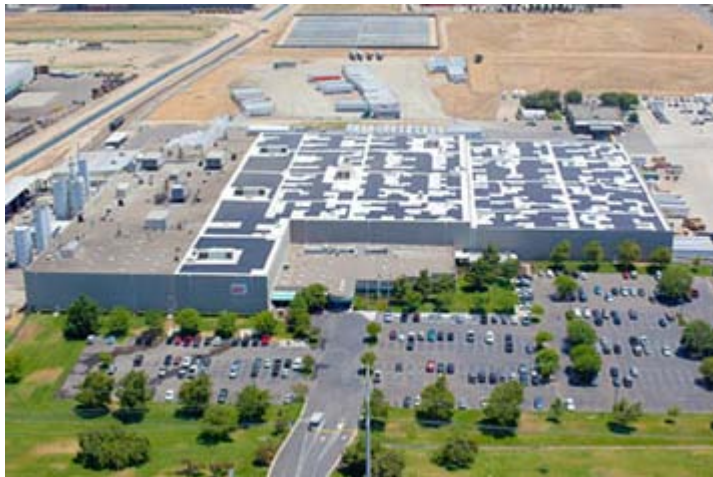
1 MW Solyndra solar panel installation on the roof of Frito-Lay's Modesto, CA plant
